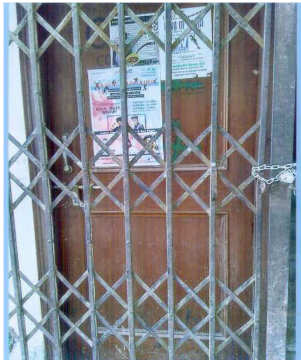
Photograph 1: Photograph of the outer metallic channel with inner wooden door - entry gate of gymnasium
